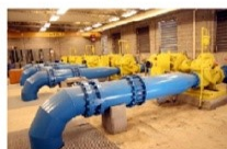
Pumping station site
