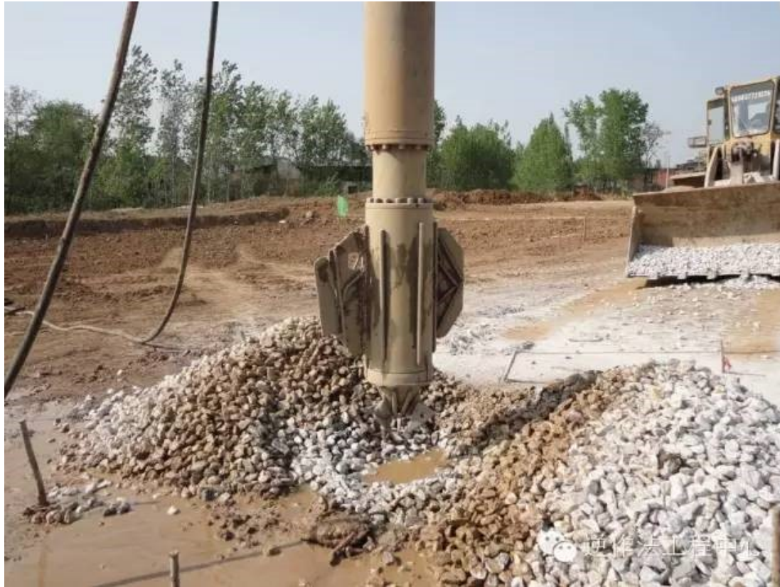
Construction of vibroflotation gravel pile
