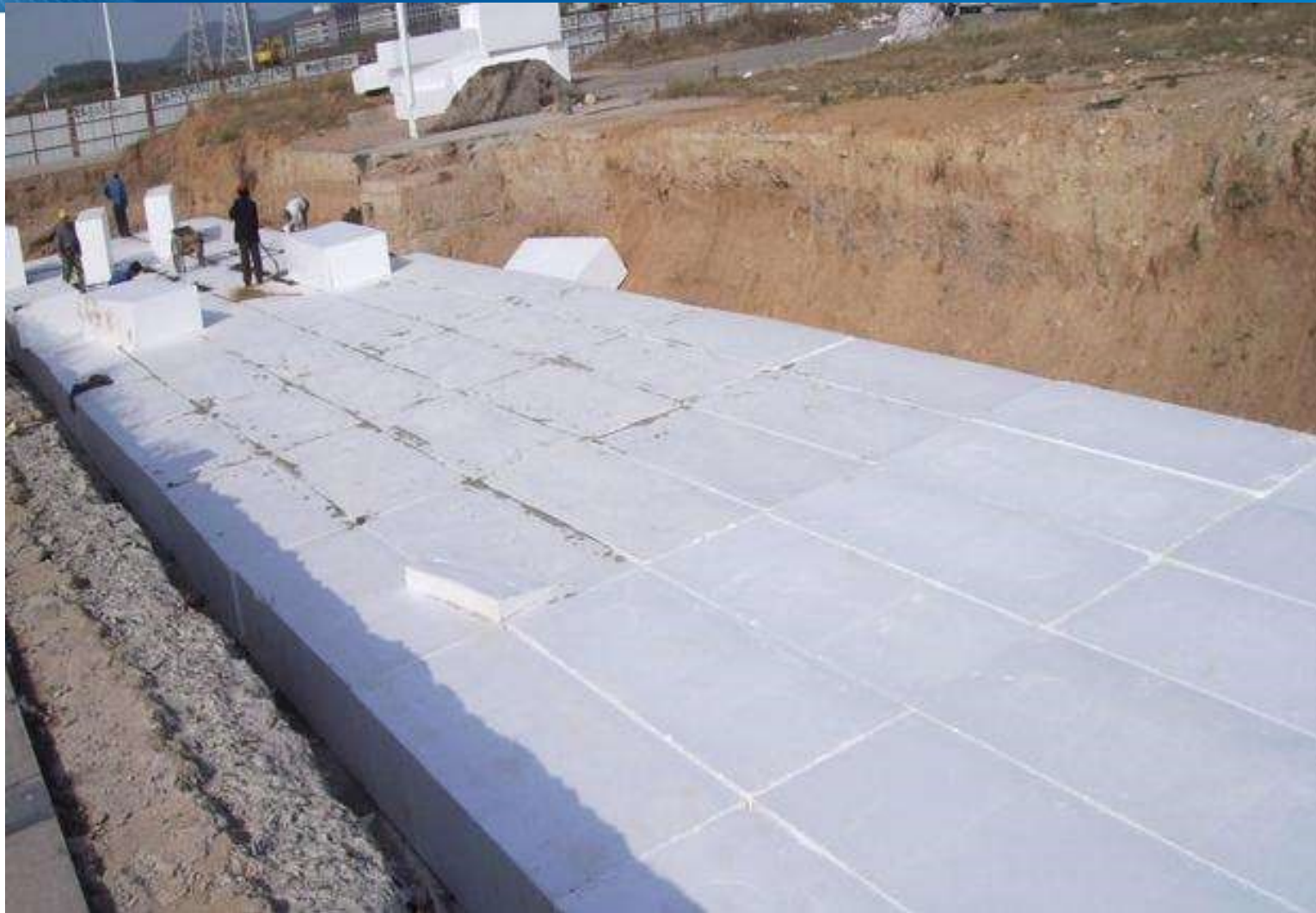
EPS super light filling method
