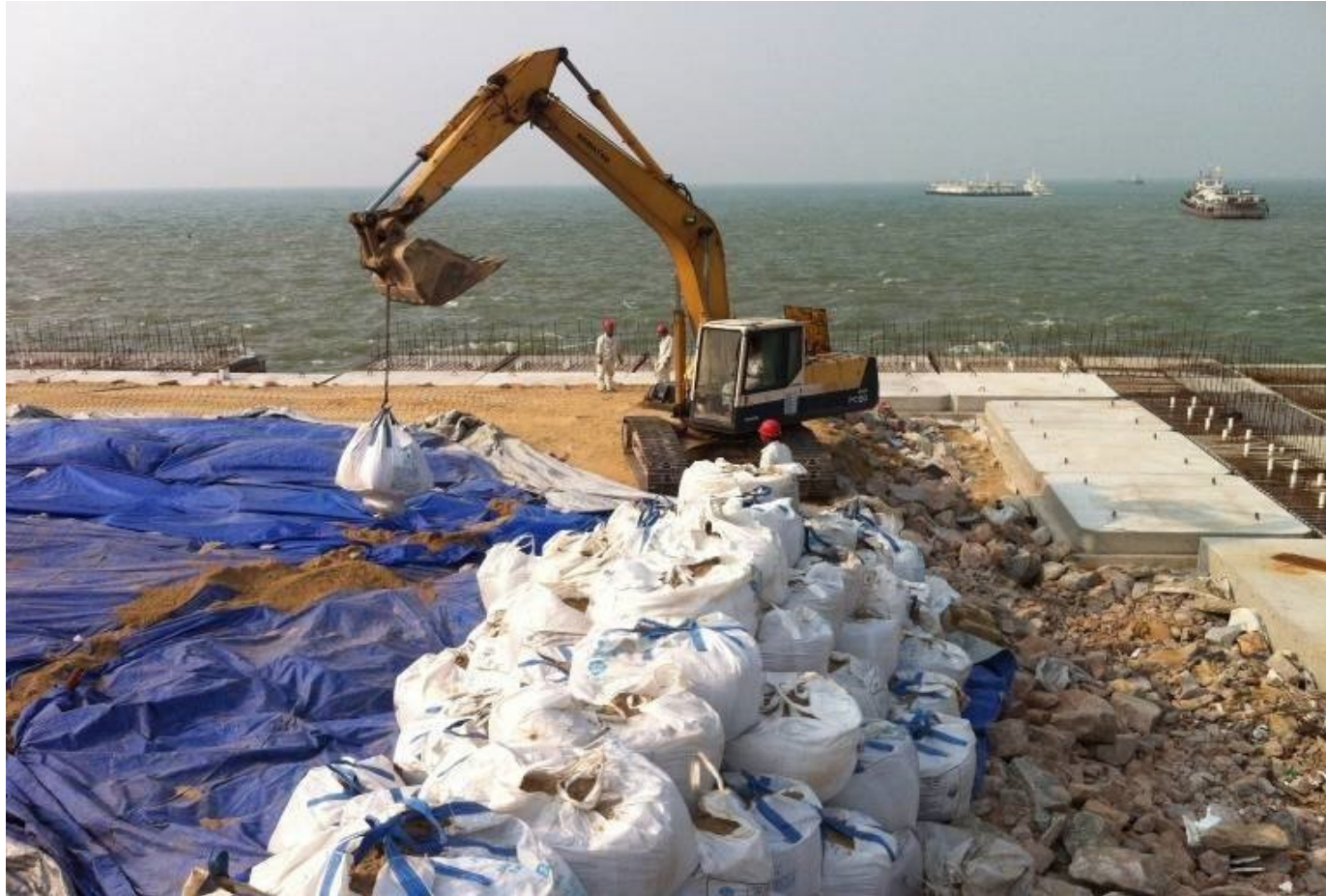
Photos of construction with preloading method
