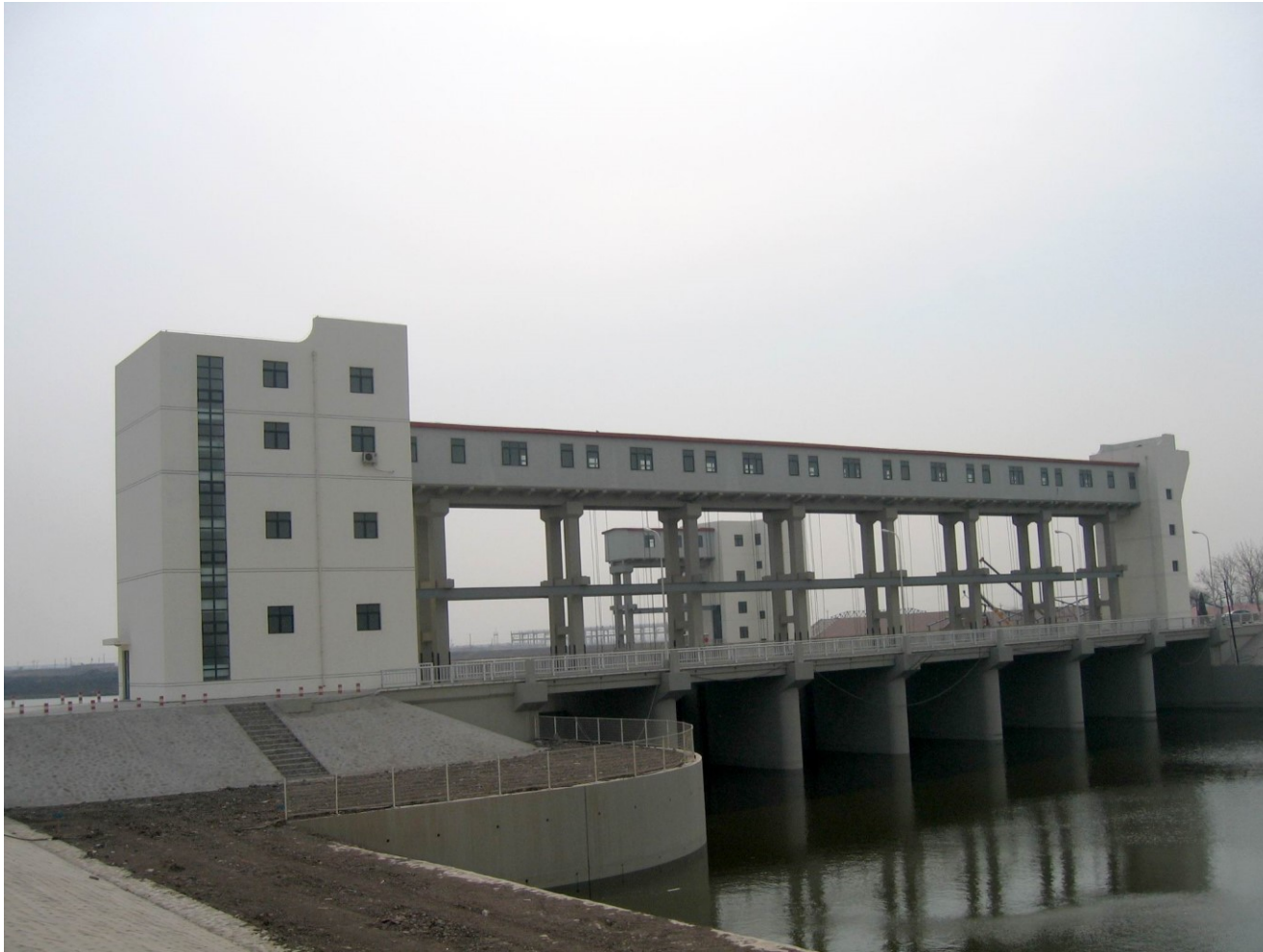
Status of Jinzhonghe Tidal Sluice
