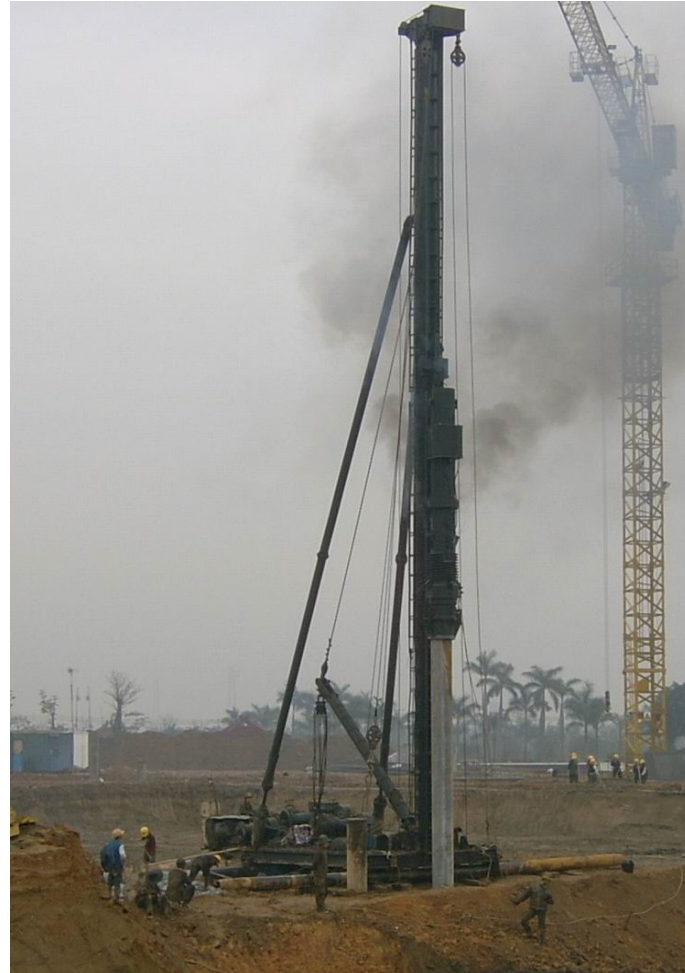
Pipe pile driving
