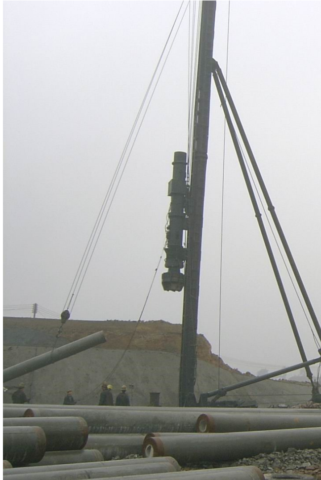
Pipe pile lifting and centering
