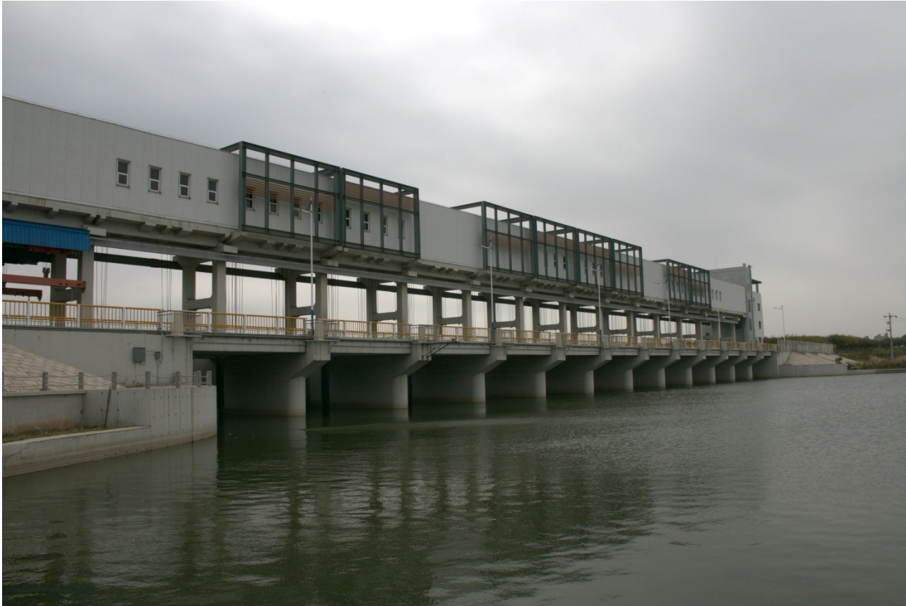
Status of Jiyunhe River Tidal Sluice
