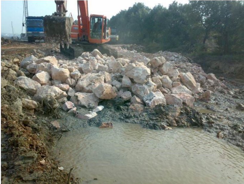
Construction of riprap squeezing method
