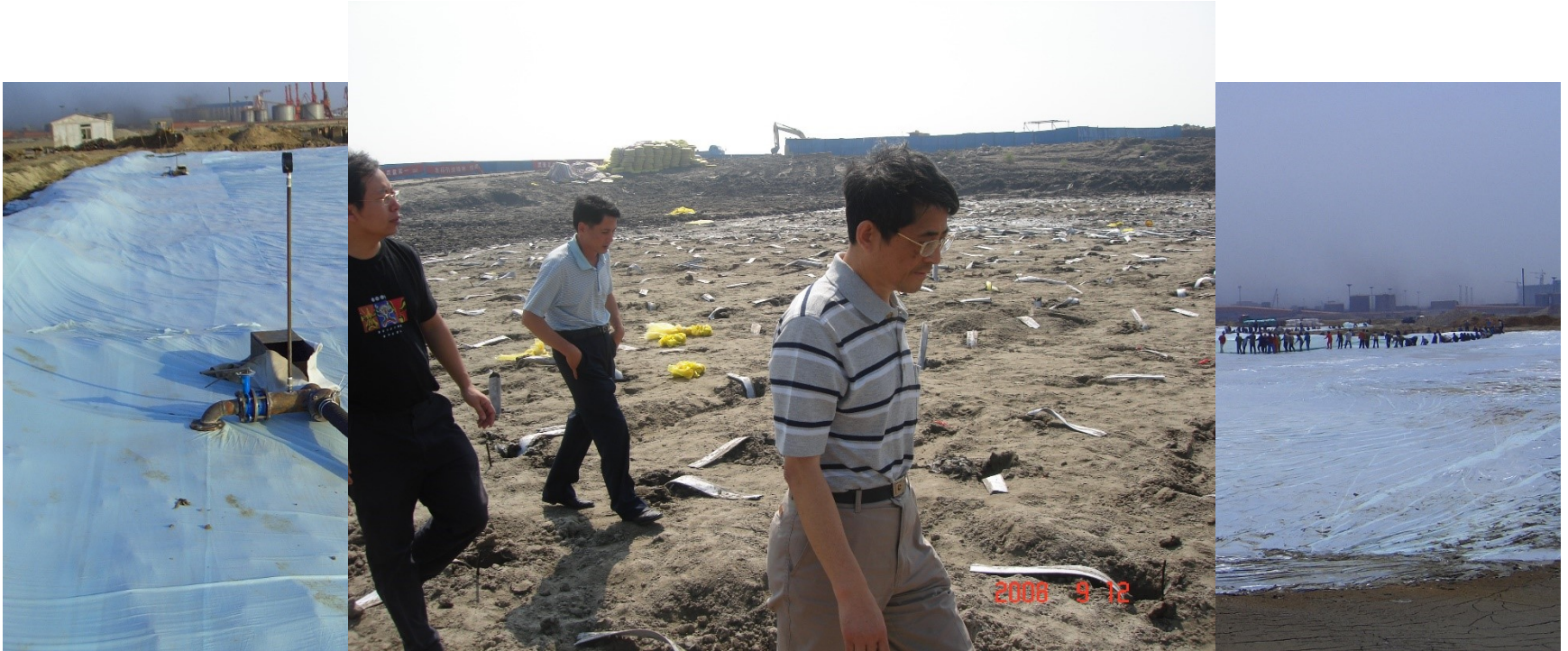
Photos of construction with vacuum preloading method in Yongdingxin River sluice
