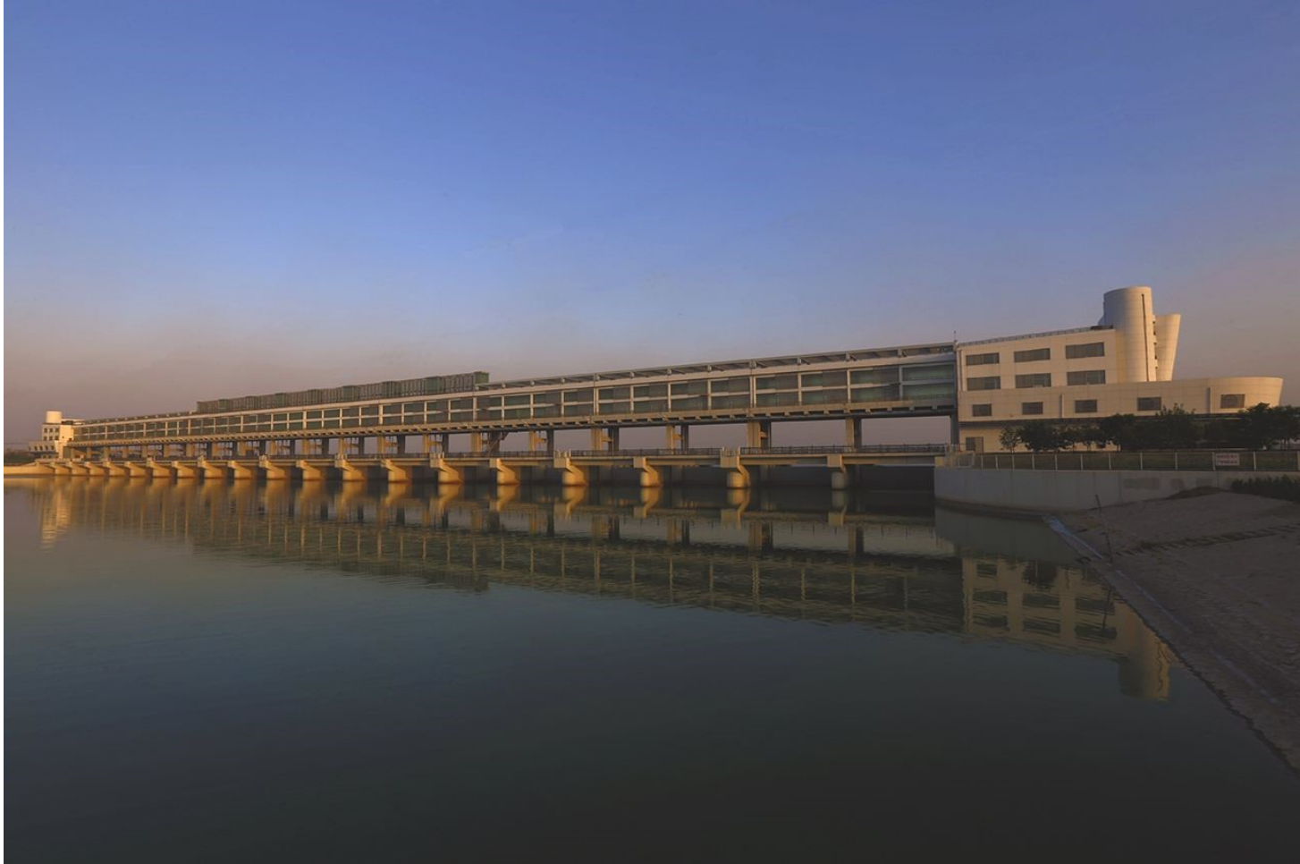
Status of Yongdingxin River sluice
