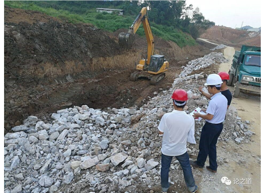
Construction of riprap squeezing method
