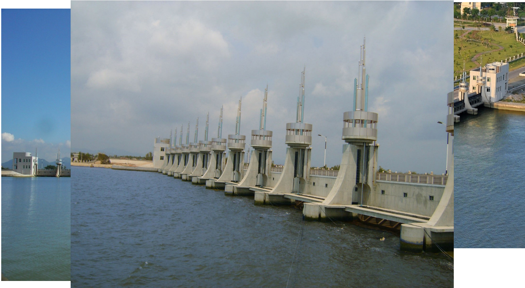
Status of Dachongkou sluice
