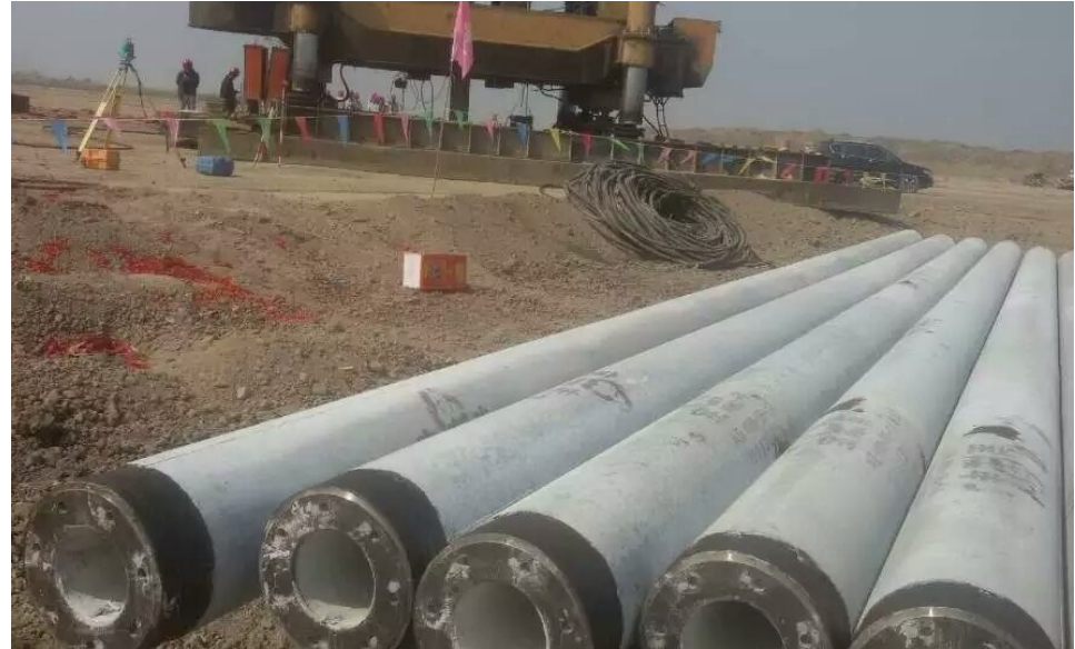
Precast concrete pipe pile
