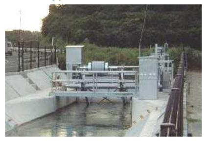
Fig.4 Mechanical Automatic Check-Gate
