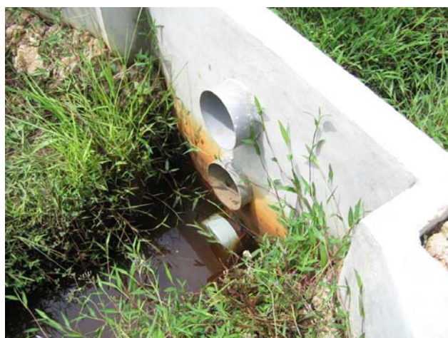
Figure 9 Water control structure in order to control upstream water level
