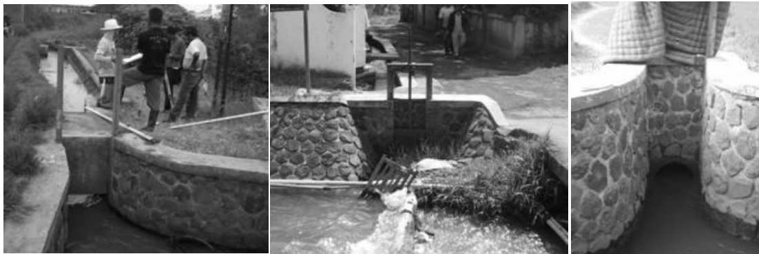
Figure 1. the Existing Condition of Division Structure
