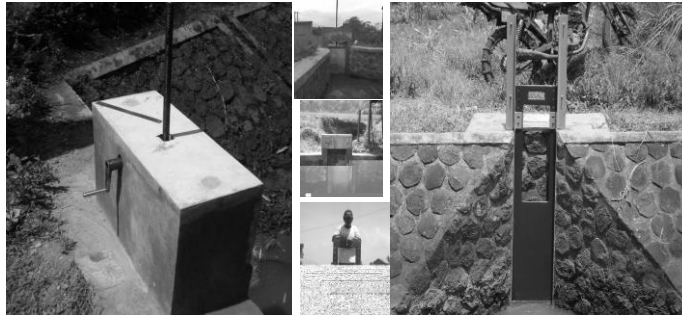
Figure 10. Application of Water Gate, Garut
